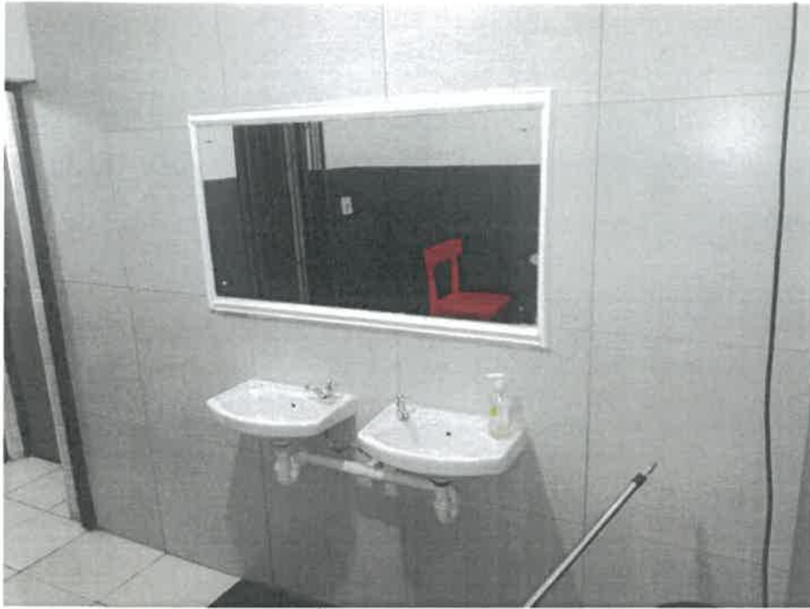
8 BATHROOM FACILITIES, MEN'S AND WOMEN'S TOILETS SEPARATED- WITH FLUSH TOILETS AND DOORS FOR PRIVACY
